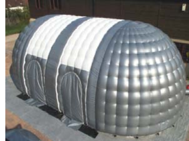
Figure 4 -Inflatable structures can be assembled easily, like the one seen above. As you can see, large volume is provided while using limited amounts of material.
